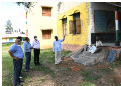
Civil Work at Govt Boys School, Tadkod
